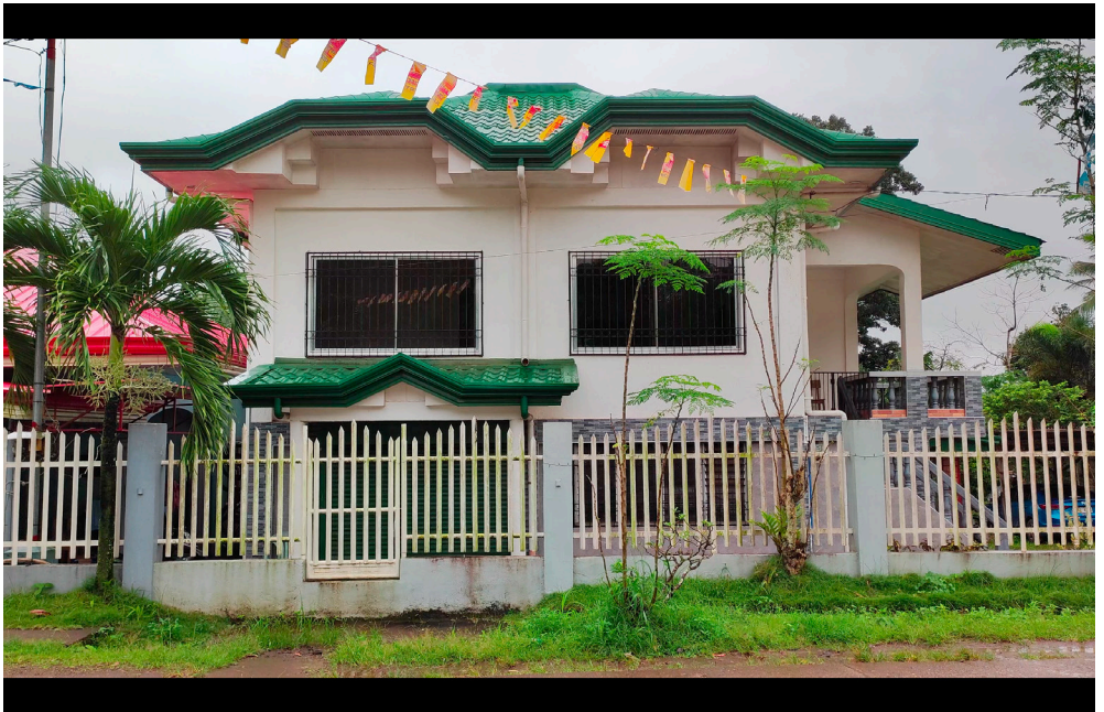
Remittance House , Sta. Agueda
