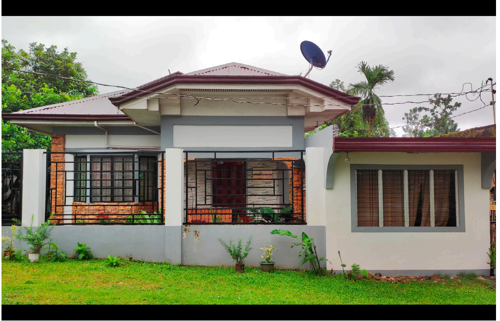
Remittance House , Sta. Agueda
