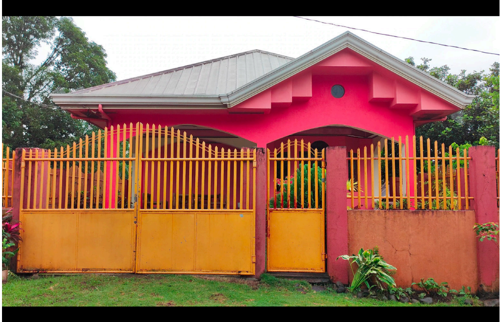
Remittance House , Sta. Agueda
