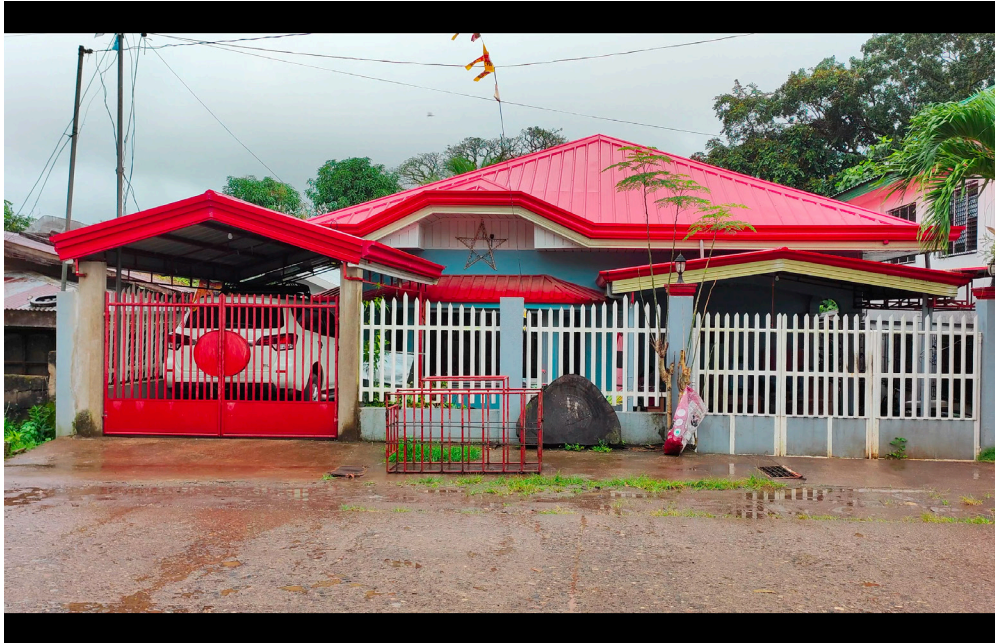
Remittance House , Sta. Agueda
